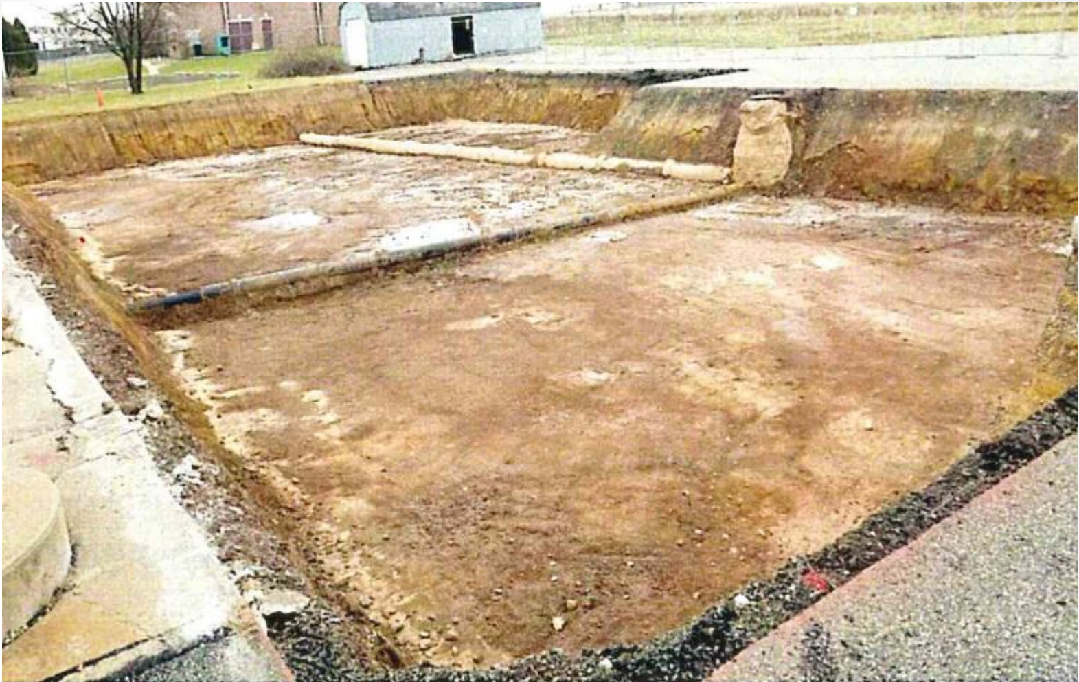
Photo shows excavation in front of Navy Fire House.
